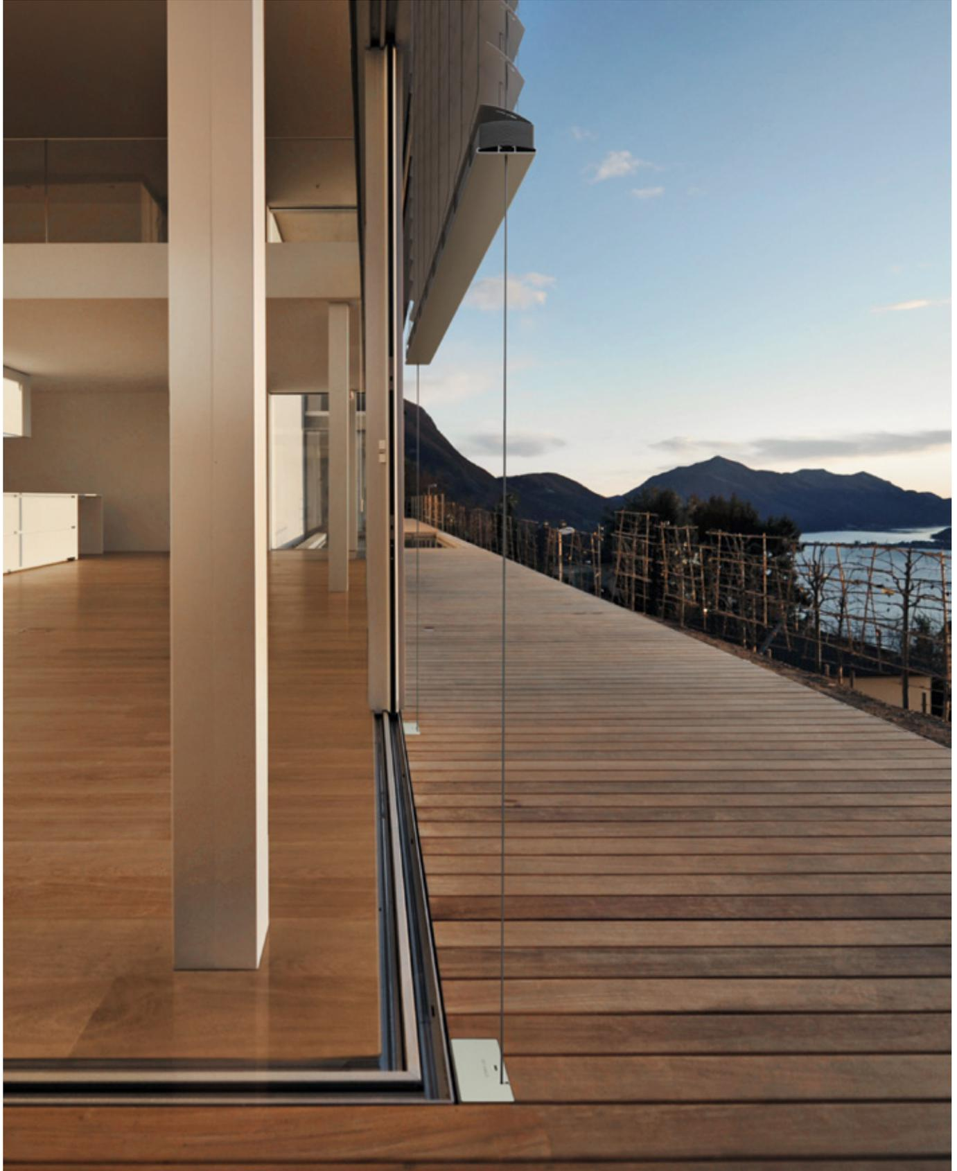
The Sun venetian blind system with its flat, 80 mm wide aluminium slats offers the perfect solar shading solution for the elegant Sky-Frame sliding windows. Slats that measure up to 3 m width and with a maximum height of 4 m are suspended on plastic-sheathed guide cords. The Sun box is recessed into the floor and the winding mechanism in the blind box facilitates swift dismantling of the guide cords to create an unobstructed opening as well as their subsequent reinstallation.
