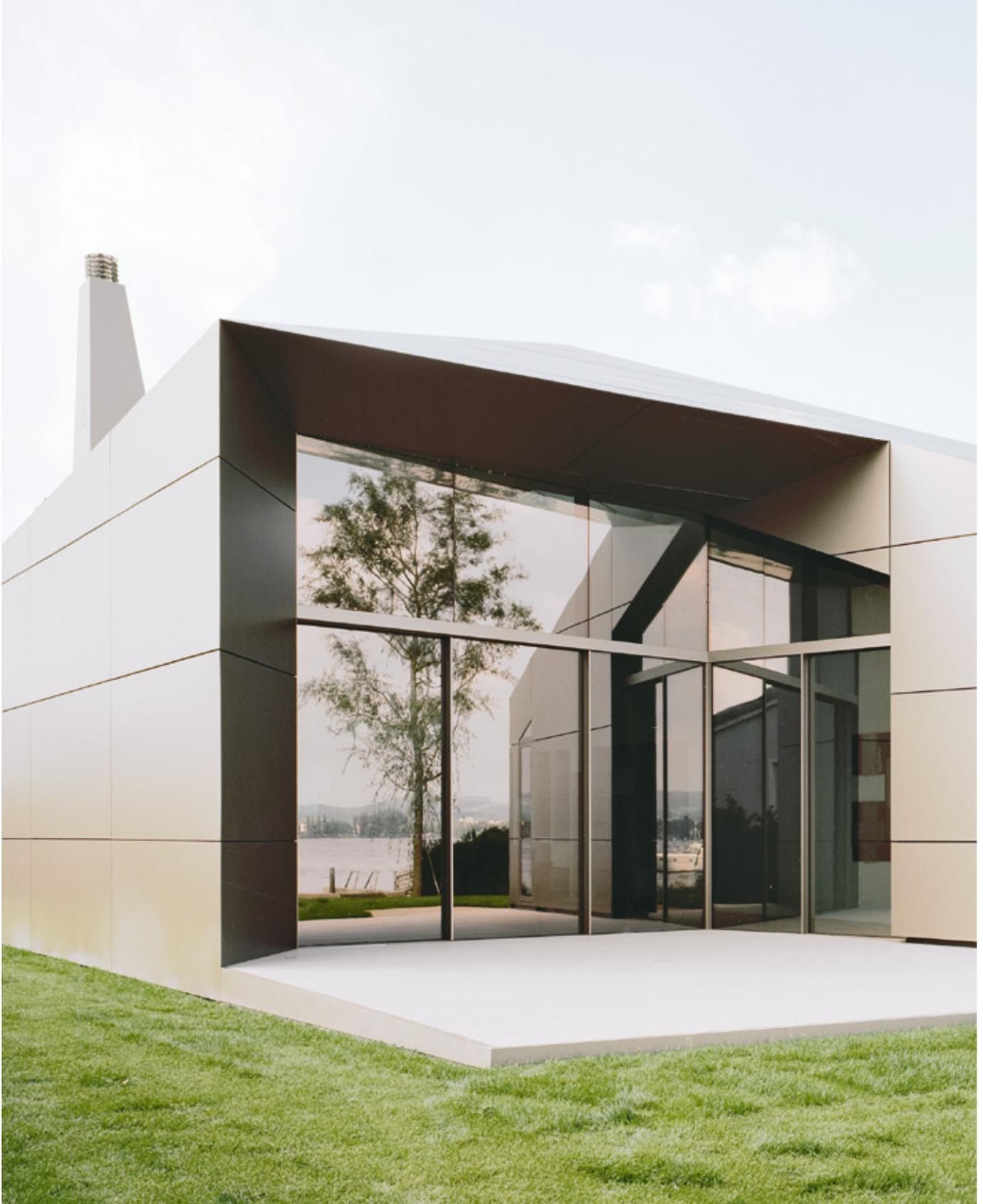
Sky-Frame Guard offers outstanding burglar resistance thanks to an adhesive bond between the insulating glass assembly and the GRP sections, as well as a multi-point locking system. Various additional components are available to meet further security requirements.
